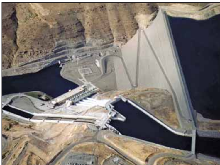
Aerial view of the Alicura project.
